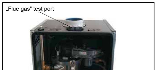
Fig.: Flue gas test with an open boiler
